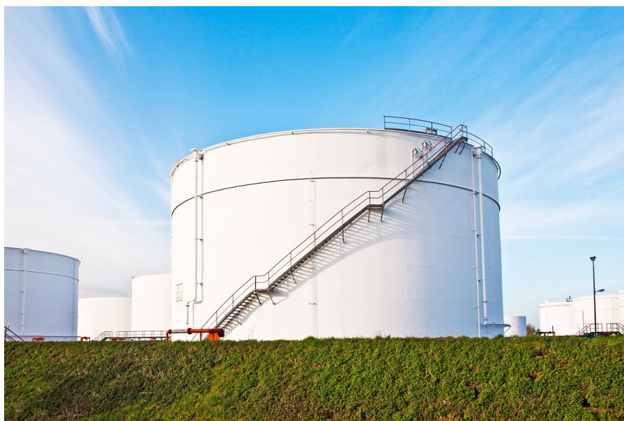
Figura 5.1: Tanques de armazenamento (Fonte: http://goodpep.com/giftforgf/wp-content/uploads/2013/10/shutterstock_50073202.jpg ).
